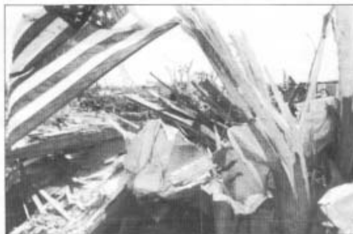
"Flag attached to a splintered tree, May 31, 1998"
